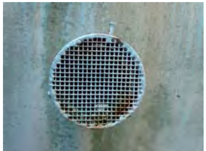
24 Unobstructed And Screened Overflow Pipe
