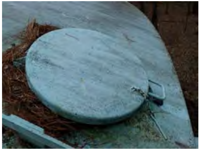
38 Hatch Closed And Secured With A Lock
