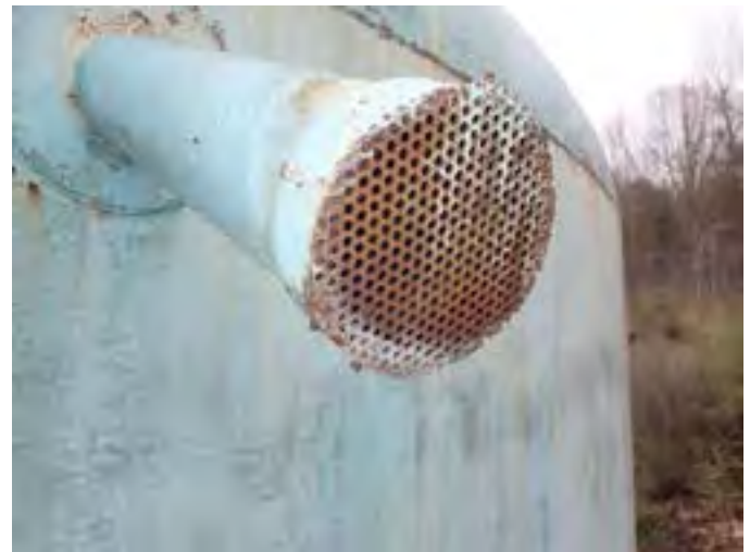
22 Unobstructed And Screened Overflow Pipe
