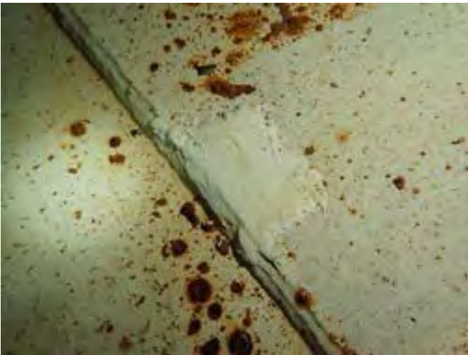
51 Additional Protective Coating Applied To The Tank Floor Having Good Adhesion Value
