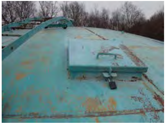
38 Closed Access Hatch Secured With A Lock
