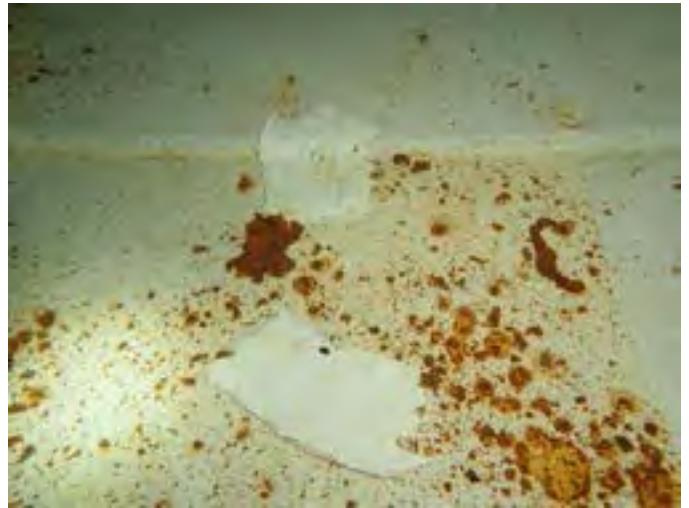
52 Additional Protective Coating Applied To The Tank Floor Having Good Adhesion Value
