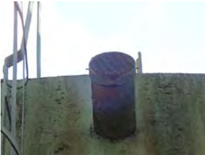
27 Unobstructed And Screened Overflow Pipe
