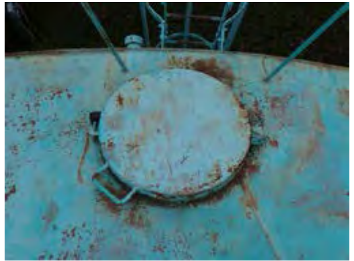
38 Closed Access Hatch Secured With A Lock
