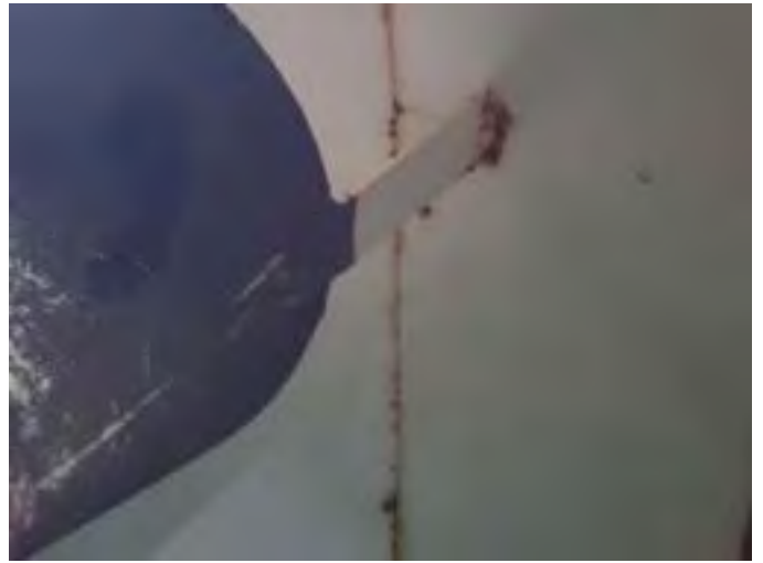
74 Overflow Pipe Supported To The Overhead
